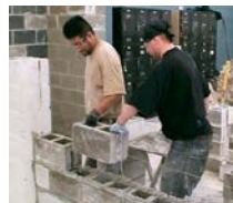
Workers use the two-mason lift technique to reduce stress of lifting and twisting.
