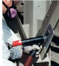
The worker at left is removing lead paint from the metal surface using a needle gun with a vacuum attachment.
