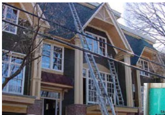
A painter was electrocuted when a metal ladder came in contact with a powerline.
